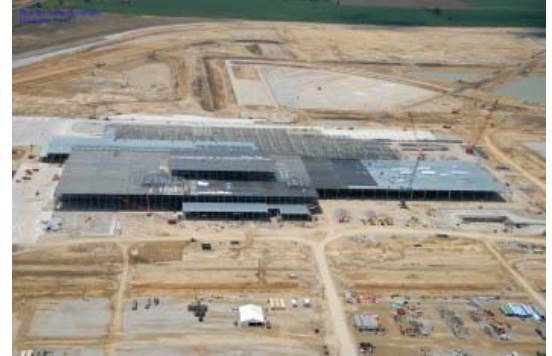
Aerial view of partially completed Honda plant in Greensburg, IN.
