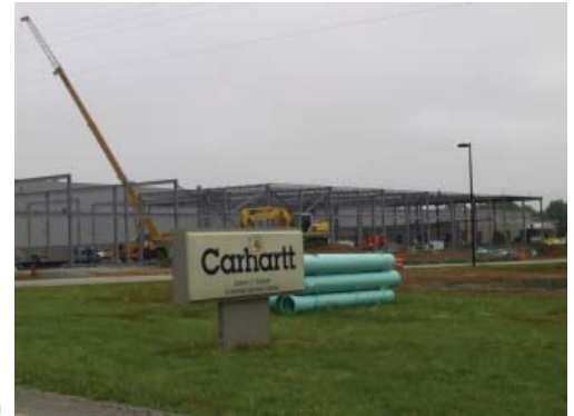
Carhartt construction site in Hanson, KY.
